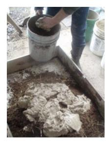
Through a long process of trial and error and advice from others, we found the quickest and easiest way to mix everything is to moisten the clay and then turn it into a thick paste without any lumps.
