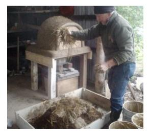
If the material used for insulation is dry, then you can get away with wetter clay.
